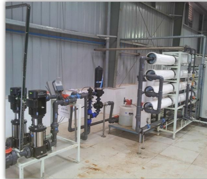
MYLAN PHARMA (UNIT 9) VISAKHAPATNAM, AP MODEL : 201 FLOW RATE : 14 m 3 /h FILTRATION GRADE : 50 MICRON APPLICATION : PRE-FILTRATION
