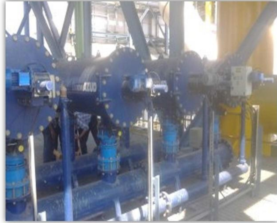
JINDAL STEEL & POWER LIMITED, ANGUL ORISSA MODEL : LXE21300 S/8 FLOW RATE : 60 m 3 /h FILTRATION GRADE : 10 MICRON APPLICATION : D.R.I PLANT (JSPL)
