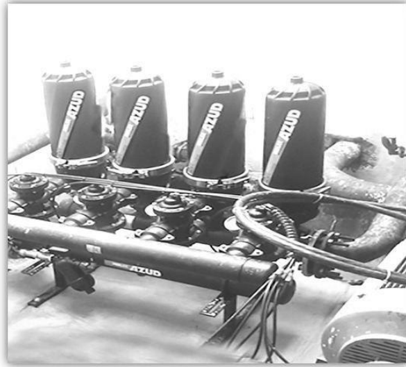
TORRENT POWER PLANT SURAT, GUJARAT MODEL : 204/6 FX FLOW RATE : 96 m 3 /h FILTRATION GRADE : 130 MICRON APPLICATION : LANDSCAPE IRRIGATION
