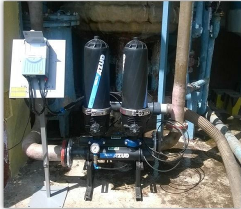
INDIAN RAYON (BIRLA GROUP), VERAVAL, GUJARAT MODEL : 202/3 FX FLOW RATE : 40 m 3 /h FILTRATION GRADE : 100 MICRON APPLICATION : PROCESS WATER
