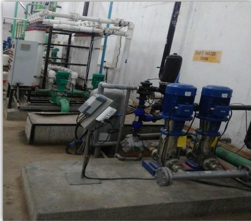
IREO TOWNSHIP GURGAON, HARYANA MODEL : 201 FLOW RATE : 24 m 3 /h FILTRATION GRADE : 130 MICRON APPLICATION : STP, TREATED WATER PLANT
