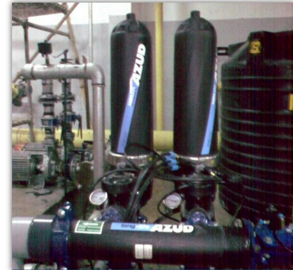
WINDMILLS LIMITED KARNATAKA MODEL : 202/3 FX FLOW RATE : 40 m 3 /h FILTRATION GRADE : 100 MICRON APPLICATION : PRE FILTRATION
