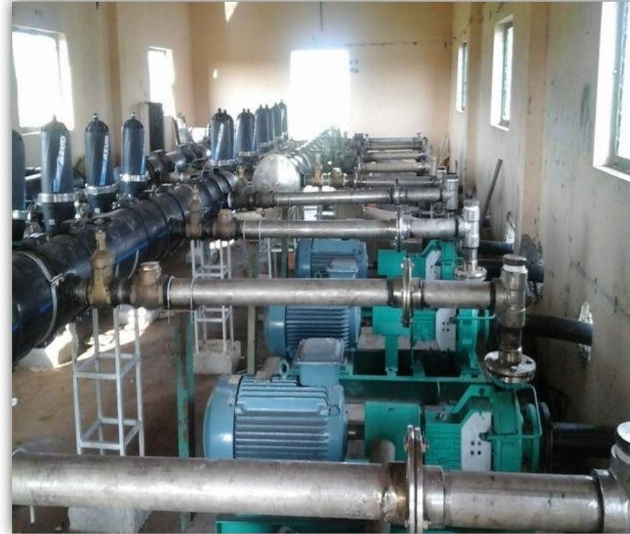
COCHIN INTERNATIONAL AIRPORT, KERALA MODEL : 16 HELIX MANUAL FILTER FLOW RATE : 128 m 3 /h FILTRATION GRADE : 50 MICRON APPLICATION : PROCESS WATER PRE-FILTRATION
