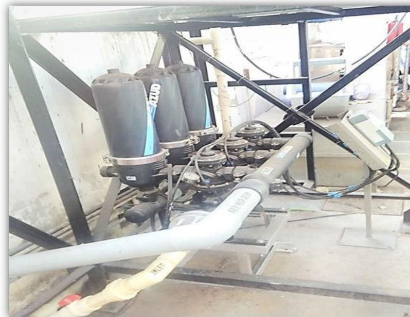
R K OVERSEAS , KIRTI NAGAR, DELHI MODEL : 203/3FX FLOW RATE : 20 m 3 /h FILTRATION GRADE : 20 MICRON APPLICATION : RO PLANT
