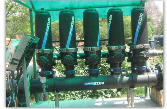
SWASTIK POLY PRINTS LIMITED, SURAT, GUJARAT MODEL : 205/4 FX FLOW RATE : 70 m 3 /h FILTRATION GRADE : 50 MICRON APPLICATION : PRE-FILTRATION
