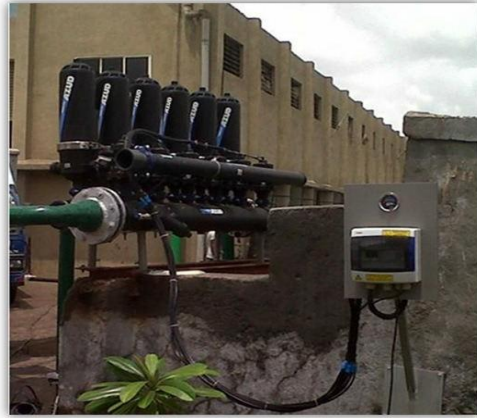
SURYODAY FASHION LTD, SURAT, GUJARAT MODEL : 208/6 FX FLOW RATE : 112 m 3 /h FILTRATION GRADE : 50 MICRON APPLICATION : RAW WATER FILTRATION
