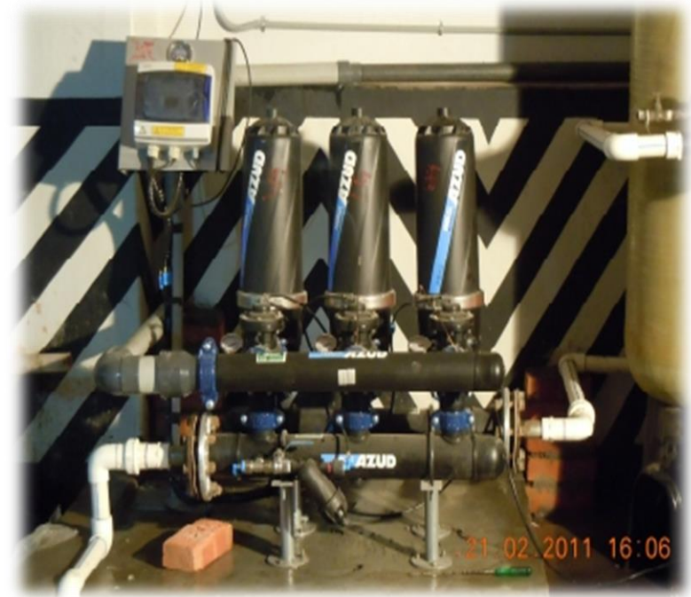
VISWARATAN HOTEL GUWAHATI, ASSAM MODEL : 203/3 FX FLOW RATE : 50 m 3 /h FILTRATION GRADE : 50 MICRON APPLICATION : WTP
